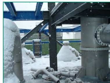
Difficult conditions for the erection due to frosty weather
