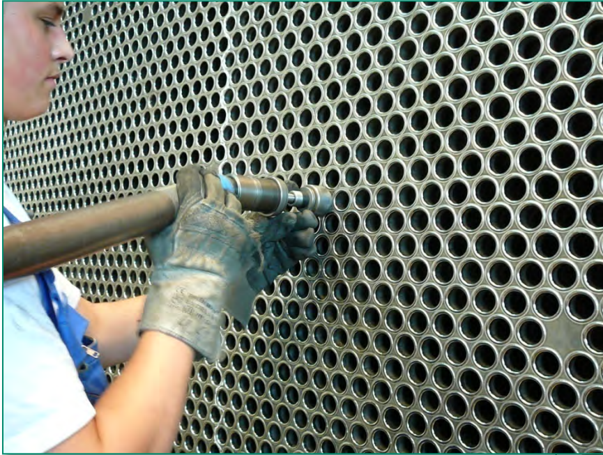
Rolling of heat exchanger tubes
