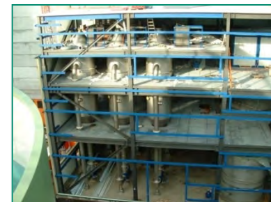
Installation is nearly finished
