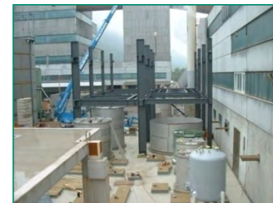
Progress of the steel structure
