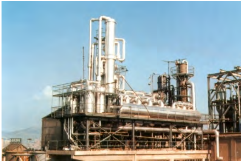
Eindampfanlage in Spanien / Evaporation plant in Spain
