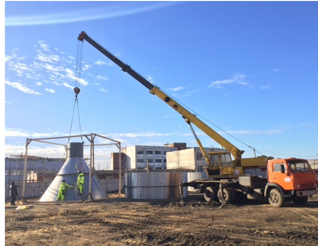
Site fabrication and mounting (Russia) Evaporating crystallizer Ø 5.400 mm, overall length 21.800 mm, 40 t, 1.4562
