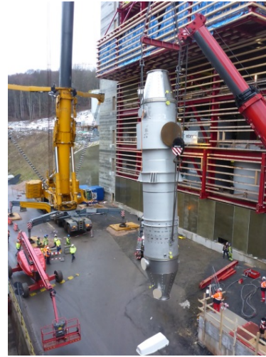
Heat exchanger Ø 3.100 mm, overall length 17.640 mm, weight 113 t A special transport on air cushions was necessary
