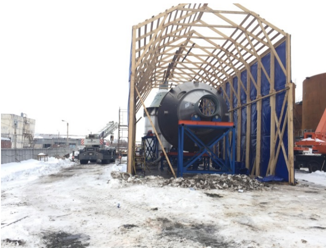
Site fabrication and mounting (Russia) Evaporating crystallizer Ø 5.400 mm, overall length 21.800 mm, 40 t, 1.4562
