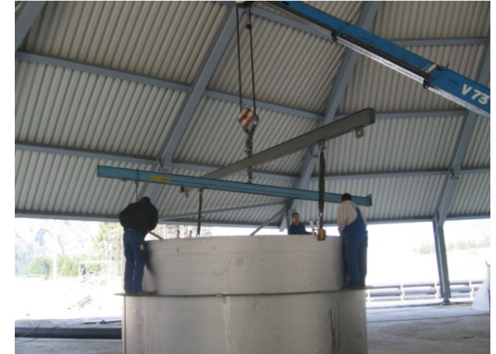
Site fabrication and mounting (Austria) Evaporation crystallizer Ø 6.400 mm, overall length 18.700 mm, 56 t, 1.4562
