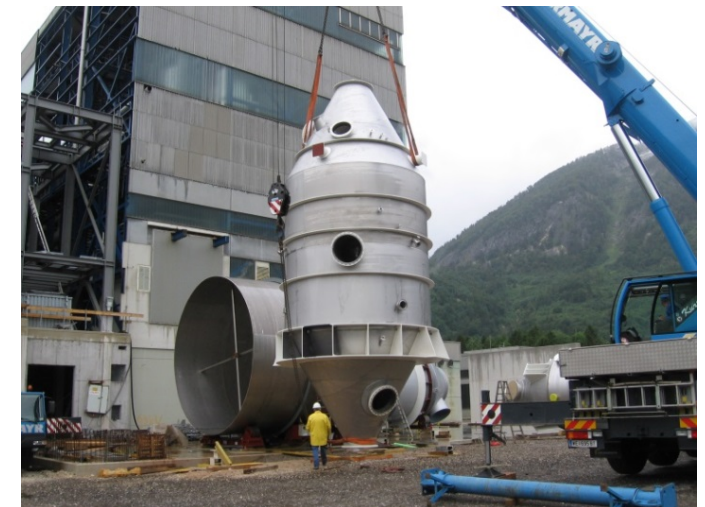
Site fabrication and mounting (Austria) Evaporation crystallizer Ø 6.400 mm, overall length 18.700 mm, 56 t, 1.4562
