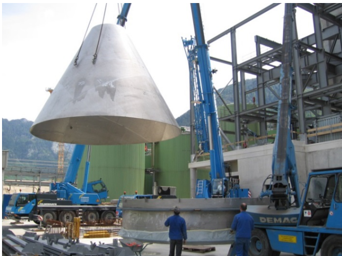
Site fabrication and mounting (Austria) Evaporation crystallizer Ø 6.400 mm, overall length 18.700 mm, 56 t, 1.4562
