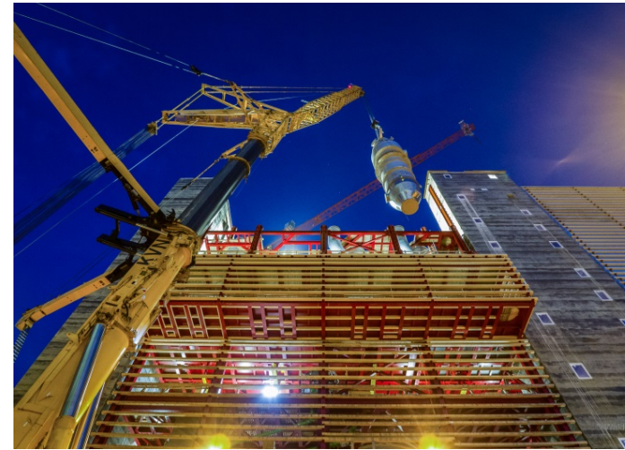
Heat exchanger Ø 3.100 mm, overall length 17.640 mm, weight 113 t A special transport on air cushions was necessary
