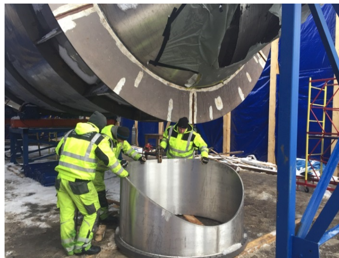
Site fabrication and mounting (Russia) Evaporating crystallizer Ø 5.400 mm, overall length 21.800 mm, 40 t, 1.4562
