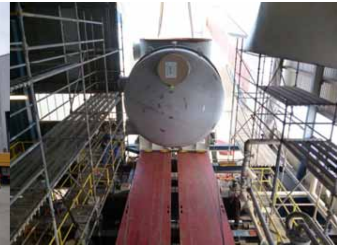
Manufacturing and mounting (Netherlands) Sea water condenser Ø 3.650 mm, overall length 10.000 mm, 40 t, 1.4462/P355GH
