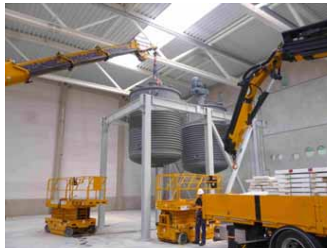
Manufacturing and mouting of agitator tanks incl. EMSR-Technology (Germany) Ø 2.200 mm - Ø 3.000 mm, overall length 5.700 mm, weight 7 - 11,6 t, Steel
